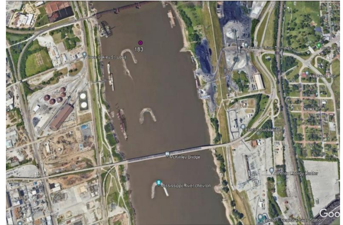
Figure 1: River Training Structures (Chevrons) located in St. Louis Harbor (Most efficient inland port #1 Dredge Maintenance location)
